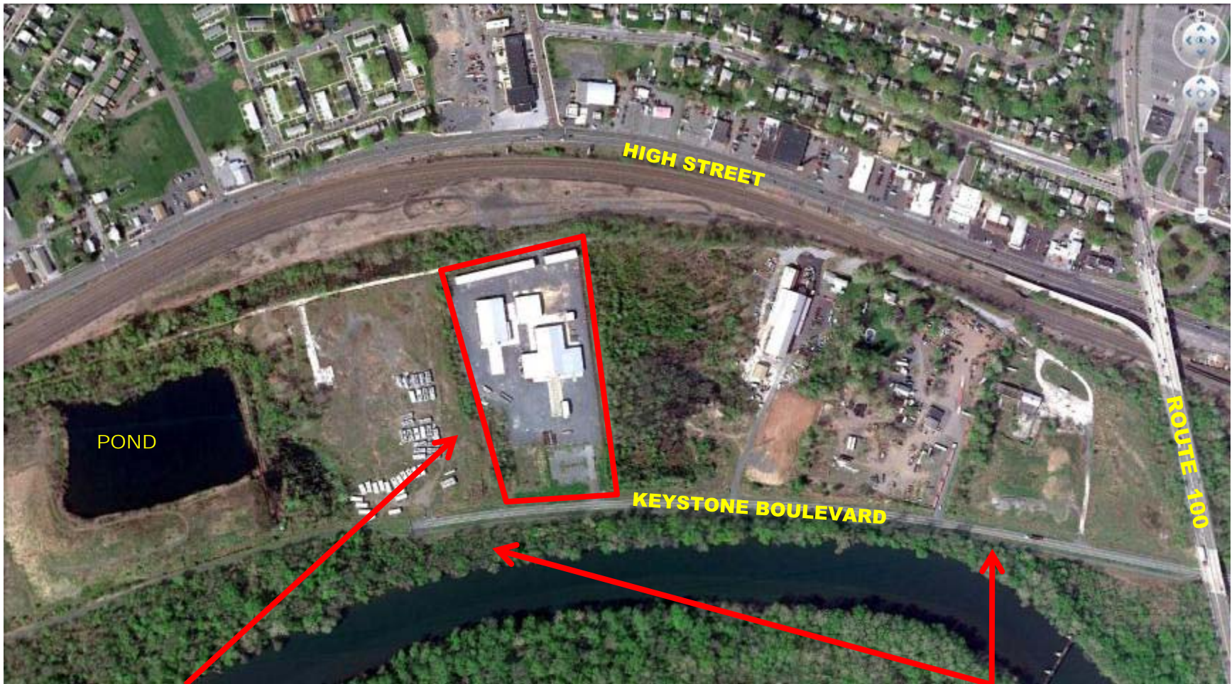
84 Lumber Co. truss plant
