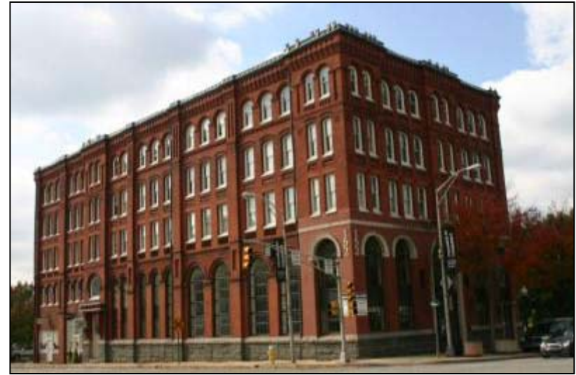
Montgomery County provided $312,000 in grant money toward the restoration of the Security Trust Building in 2002.
