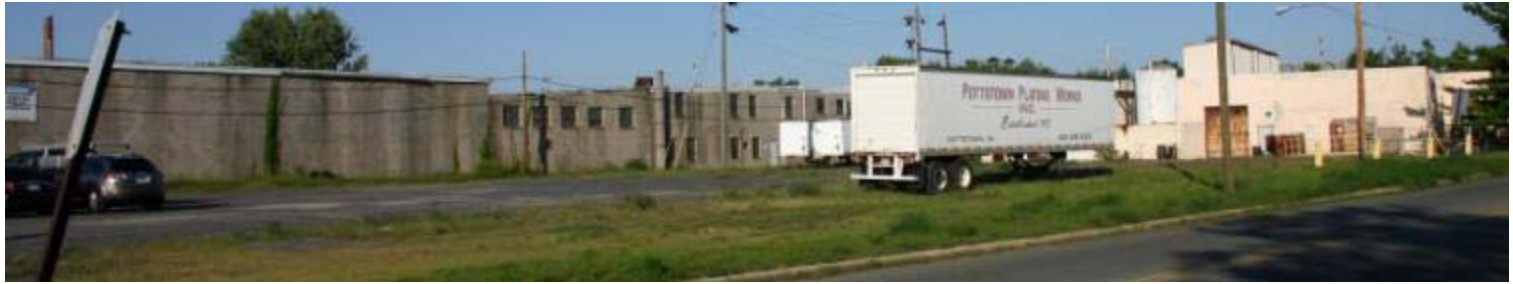
Pottstown Plating Works, right
