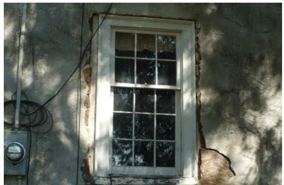
Side Elevation window frames (and sashes) have been replaced, and are ill-fitting.
