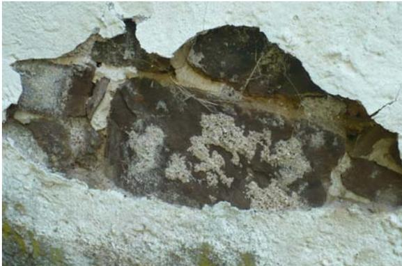
Pointing mortar remaining beneath stucco indicates original ridge-pointed condition.
