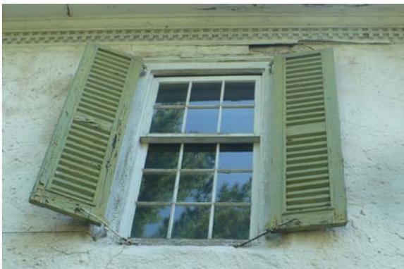
Front Elevation window frames remain intact and fit well, sashes are replaced.
