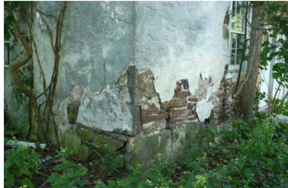
Some exterior movement of stone and rising damp is apparent.
