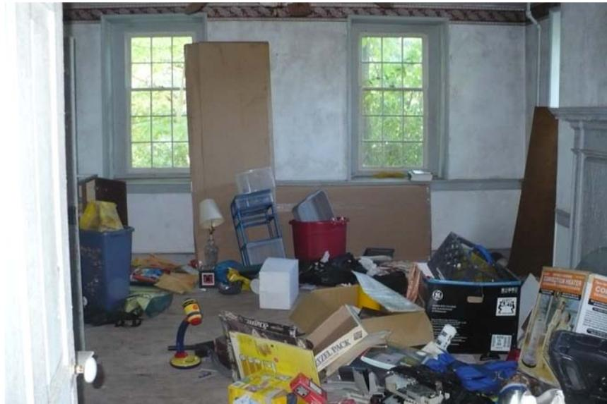
Typical First Floor Parlor looking West; note continuous chair-rail, intact wood window moldings, original fireplace mantel at right. Ceiling height is 8'-4".
