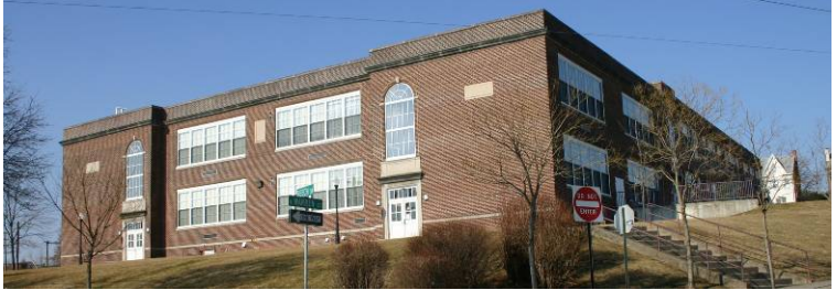
The Jefferson School was sold in 2002 to Pennrose Properties for $400,000, which converted the school into 46 apartments.
