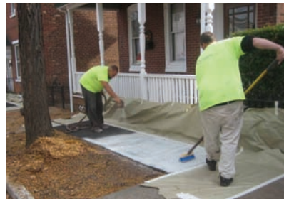
Asphalt is used for the Schuylkill River Greenway, left, and the Hill School quad, below left. Trees Inc. recently replaced 14 lifted sidewalks on Walnut Street with asphalt, then covered it with a permanent concrete-colored epoxy solution.
