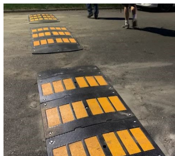
ABOVE , speed "humps" in Detroit have gaps to allow emergency vehicles to pass through unimpeded.
